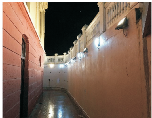
Fig. I.2.6: Retaining wall after renovation.
