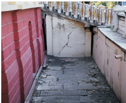
Fig. I.2.5: Side view of entrance staircase.
