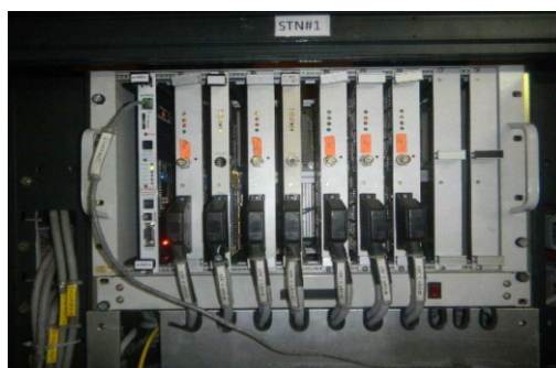
Fig. A.11.2: mVME2c controller board installed in Indus-1 LCW plant control system for field testing.
