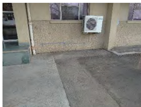
After cleaning outside front door of Block G
