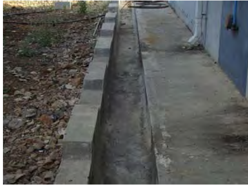
After cleaning – Trench line
