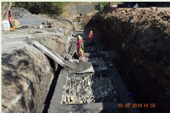
Fig. 32 Reuse of construction debris: Retaining wall for the FEL laboratory extension (1/2).
