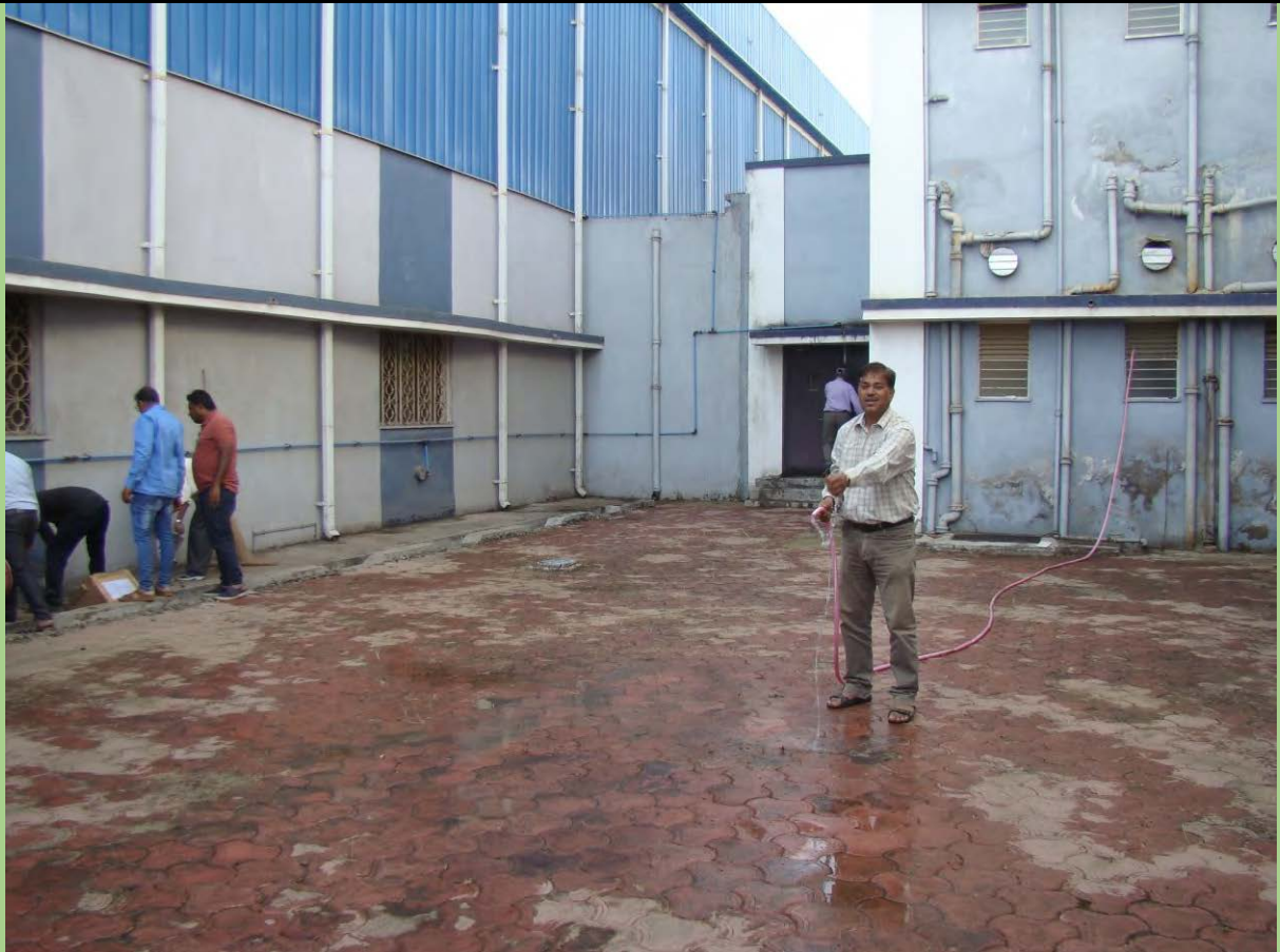
Final cleaning and washing of cleaned area
