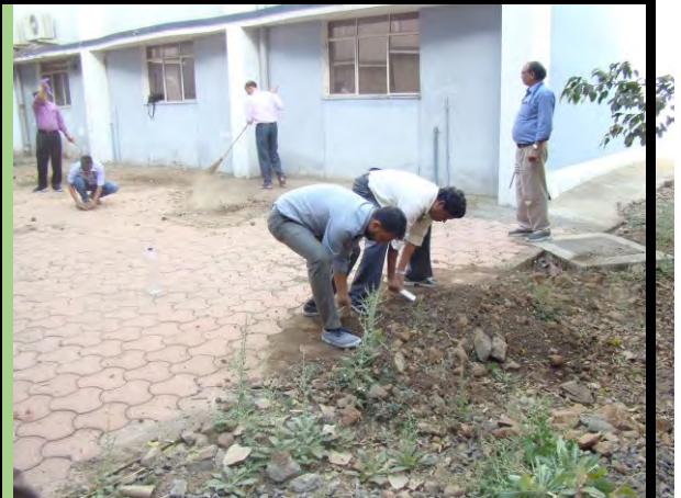
Removal of rocks and soil from the floored area
