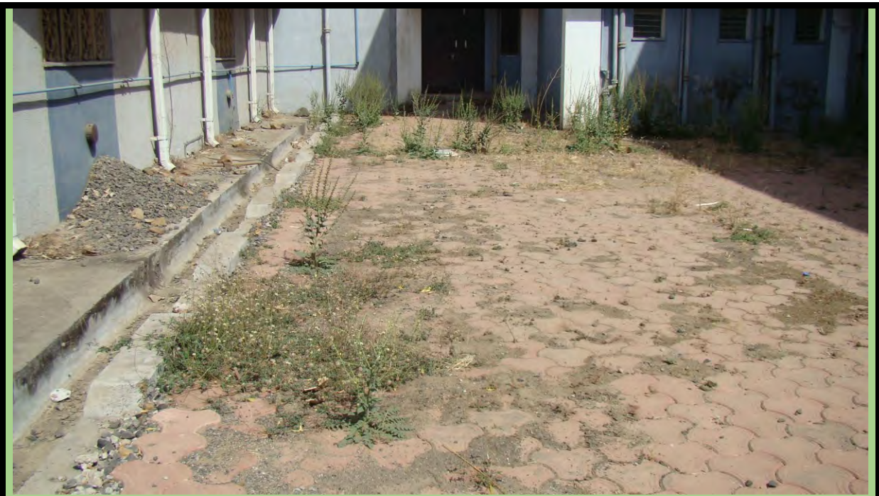
Back yard of SCRF building (Before cleaning)
