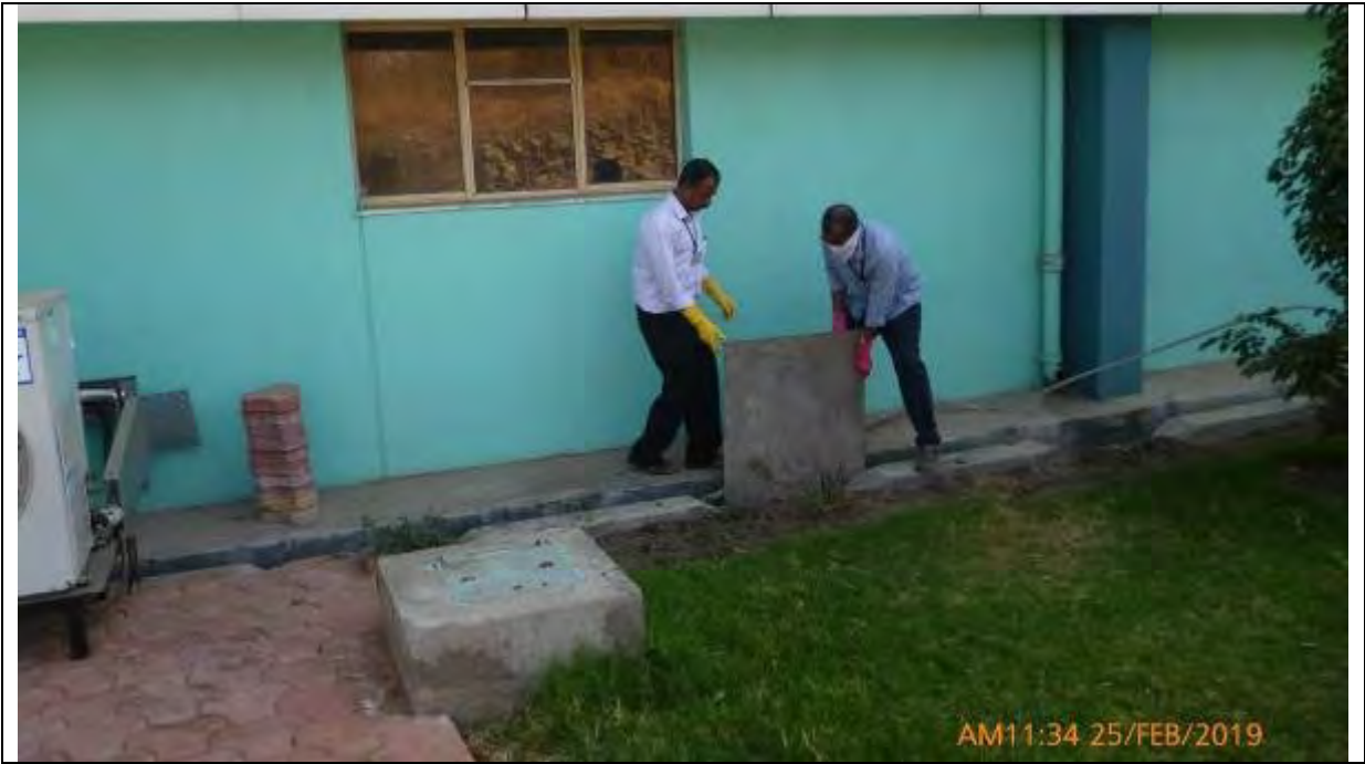
PLDD staff members cleaning west side of H ion building
