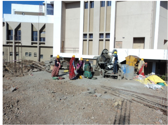
Central complex site
