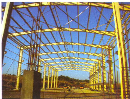
Fig. I.5.1 View showing the erection work in SCRF laboratory
