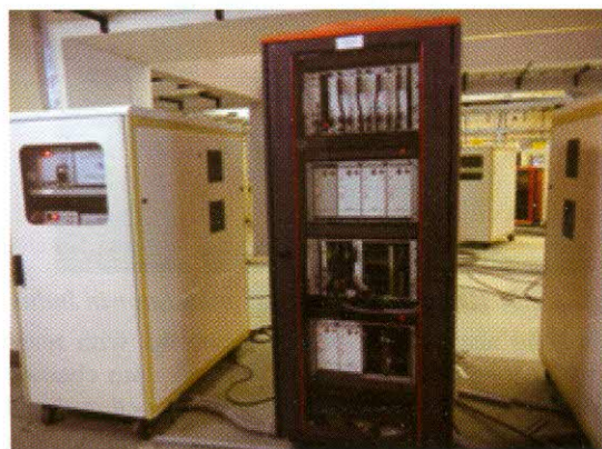
Fig. A.3.1: Equipment Control Station for Active Shunt Power Supplies for BBA in Indus-2
