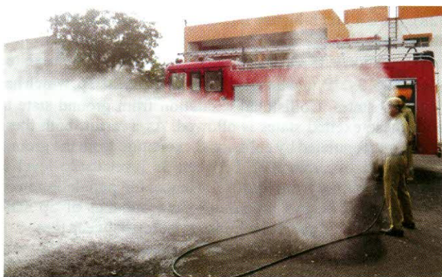
Picture I.3.3: The water mist system in operation
