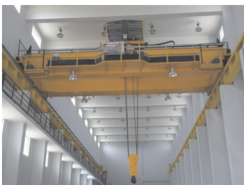
Fig.I.2.1: 50 MT EOT Crane installation at MTL Lab.
